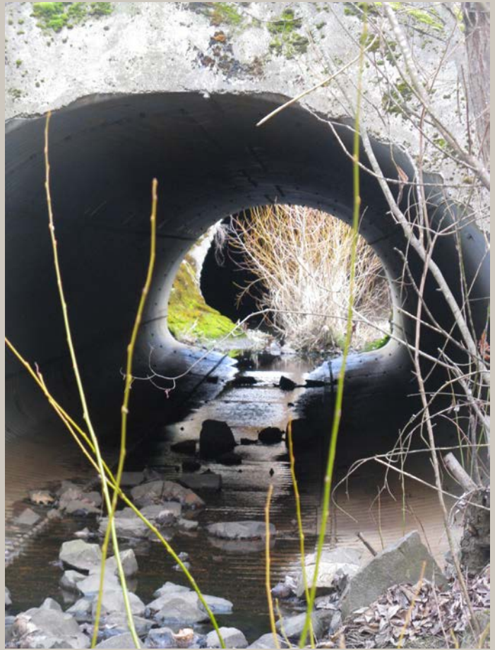
The Mill Race runs under several culverts in South Town.
